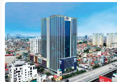
VINACONEX DIAMOND TOWER
